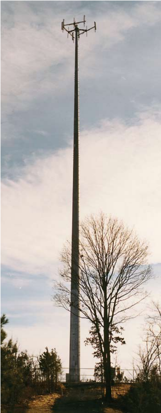
Every tower section and steel fabricated component is hot-dipped galvanized after fabrication for long-life protection against environmental corrosion damage.
